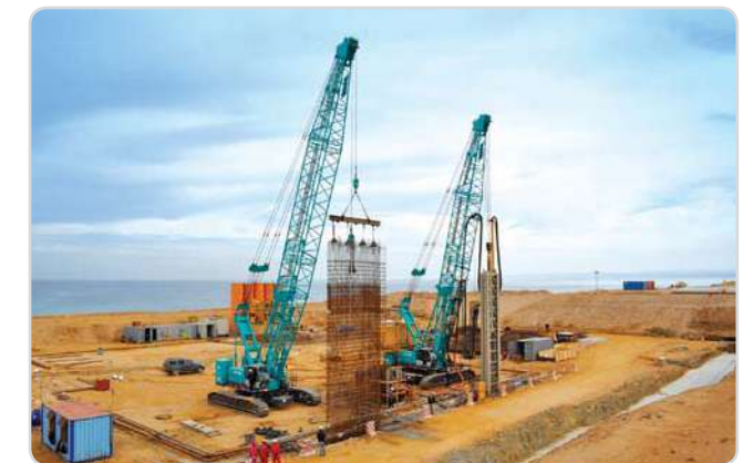
Placing of Steel Reinforcement
