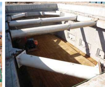
Algeria Oman Fertilizer Plant Outfall (ALGERIA) · 굴착깊이 : 11.9m · PPS 직경 : ø 800mm / ø 1,000mm
