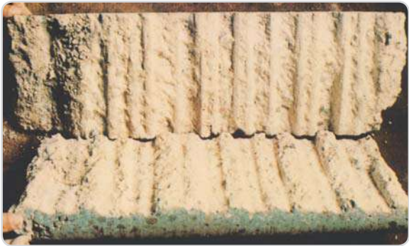
Detail View of Joint
