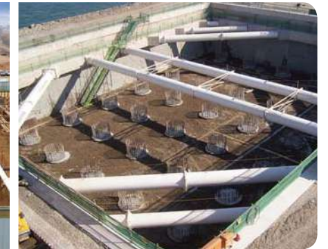
North Port Bridge Marine Special Foundation, Busan · PPS installation layer & length : 1 layer / 250m · PPS diameter : ø 1,200mm
