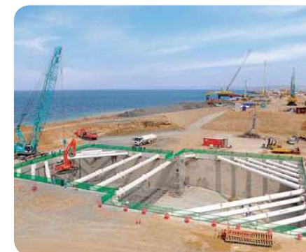
Algeria Oman Fertilizer Plant Intake (ALGERIA) · 굴착깊이 : 10m · PPS 직경 : ø 800mm / ø 1,000mm
