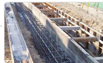
Placing of Steel Reinforcement
